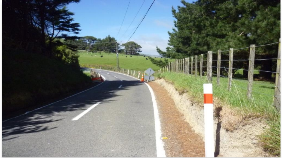
Photo 1: Existing Ohariu Valley Road Prior to Upgrade – Southern end. Note two-way provision and substandard lane width.
