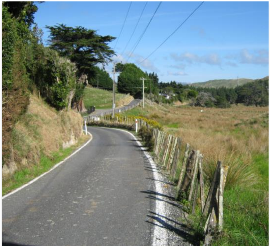
Photo 2: Existing Ohariu Valley Road Prior to Upgrade – Northern end. Note single lane provision and reduced sight distance.
