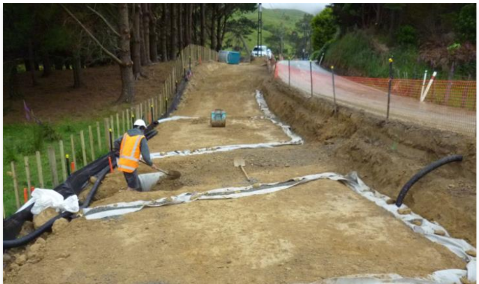
Photo 4: Ohariu Valley Road during reconstruction. Note dedicated live traffic lane and construction working zones.
